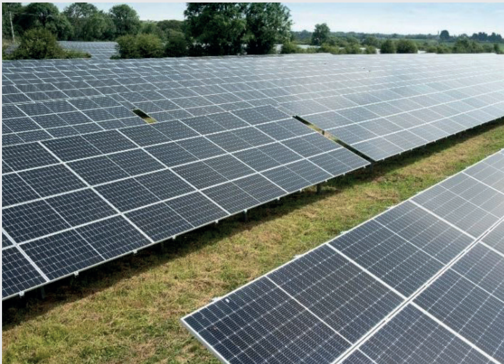
Photo: Image courtesy of Enerpower www.enerpower.ie
